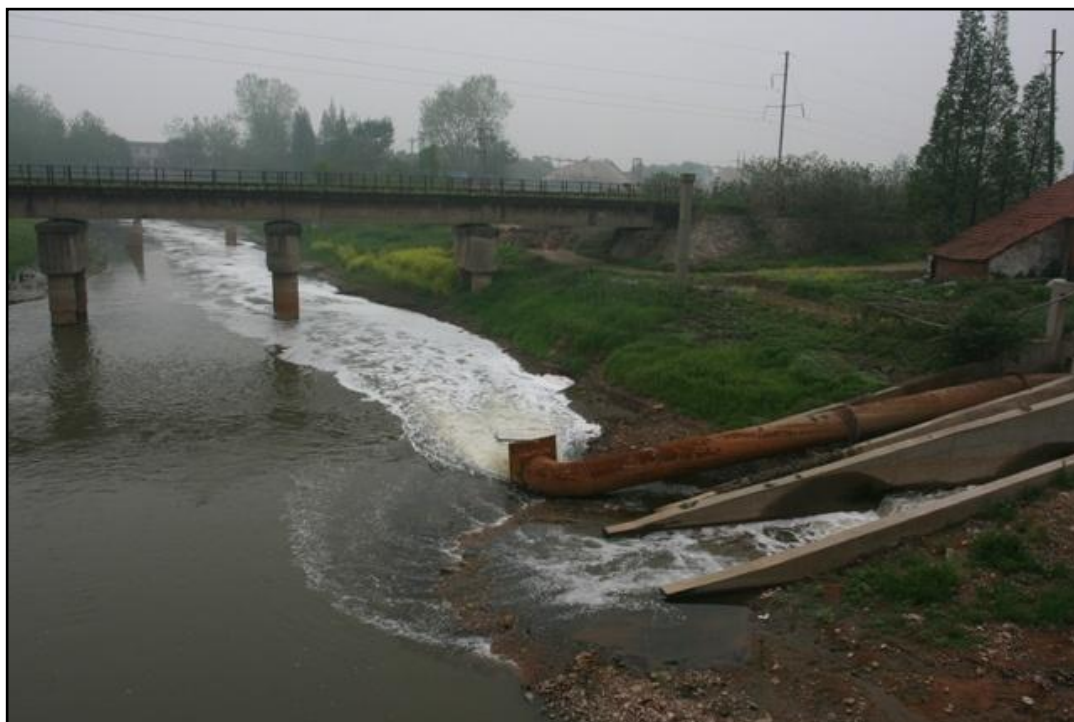
Figure 8: Discharge Outlet Used by Meiko Electronics & Chenming Paper Companies, Photo: Ma Jun
