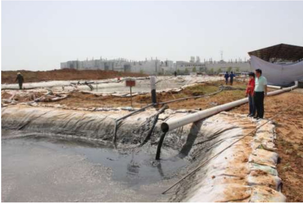
Figure 17: Nantaizi Lake Site Works
