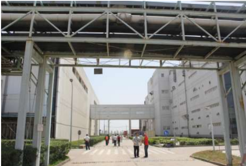
Figure 7: To avoid the mixing of wastewater and storm water, the pipes that carry industrial wastewater that were previously underground have been moved above ground.
