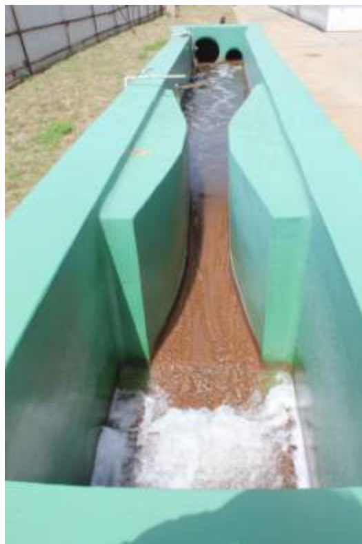
Figure 11: Final Discharge Outlet for Production Wastewater
