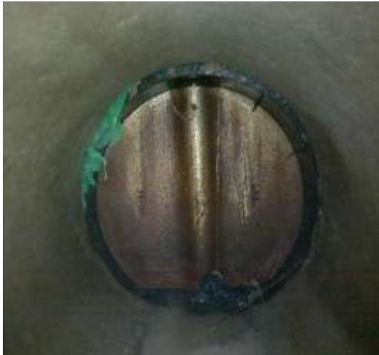
Figure 8: Storm Water Outlet with Tamper Proof Seal
