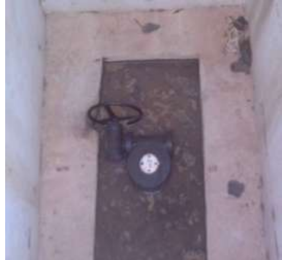
Figure 8: Storm Water Outlet with Tamper Proof Seal
