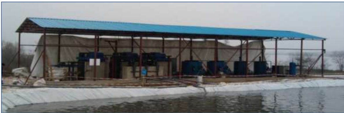
Figure 13: Sedimentation pools and centrifuges at the Nantaizi Lake site
