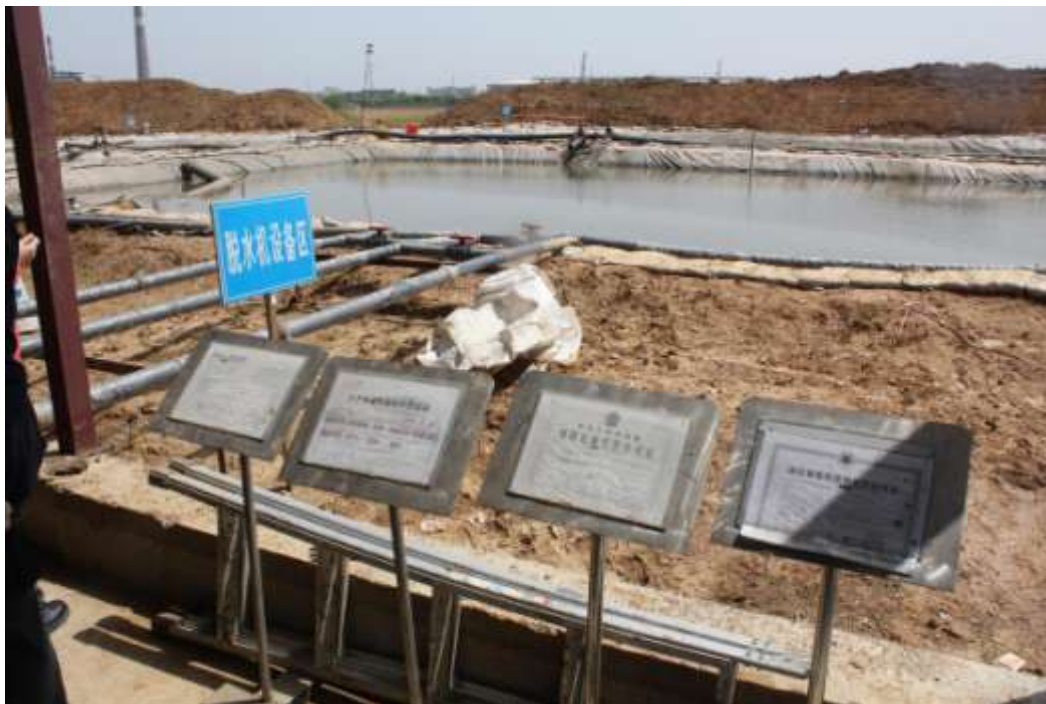
Figure 16: Nantaizi Lake Site Works
