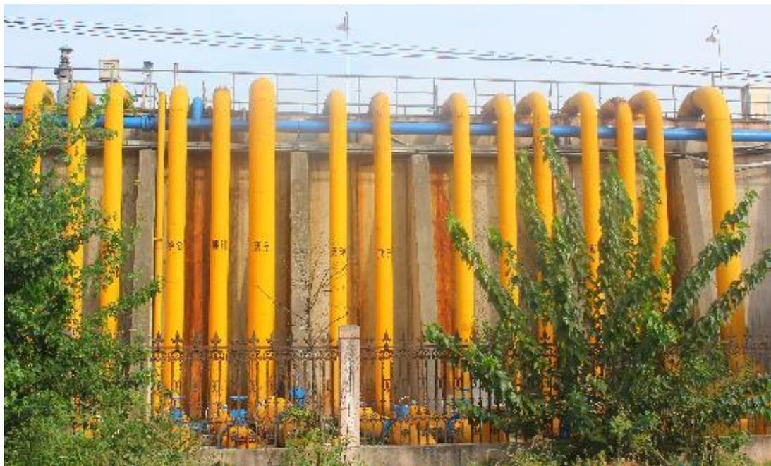
Fig 14 Wastewater influent pipes from each company that discharges into the Dangwan Wastewater Treatment Plant
