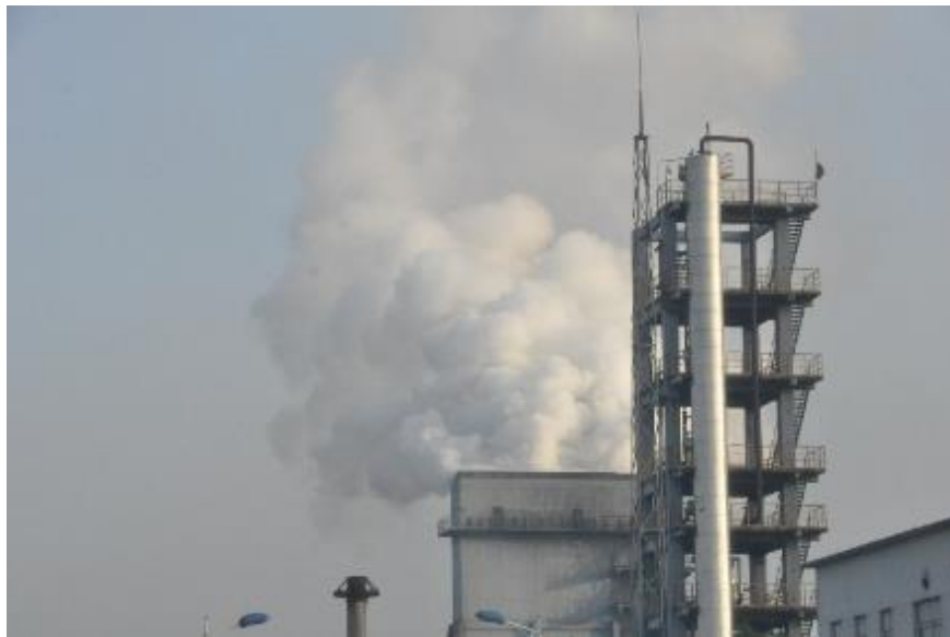
Figure 26. Flue gas emitted by the wet coke quenching tower of Sinochem Zhenjiang Coking Co., Ltd. (picture taken by Lvse Jiangnan on July 9, 2014)
