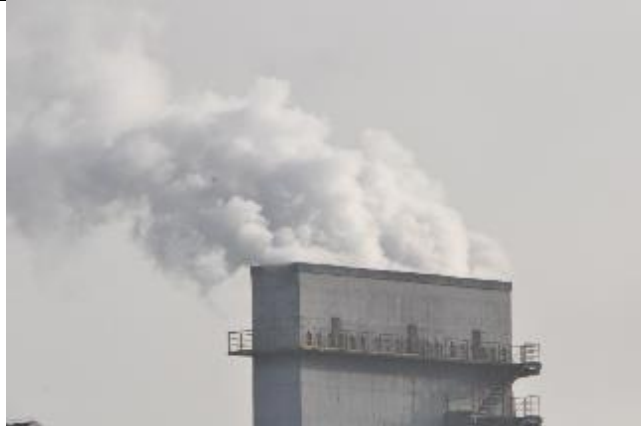
Discharge Outlet of the Flue Collector (wet quenching tower)
