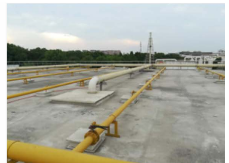
► Figure 5 Upgrade of the WWTP odor collection systems
