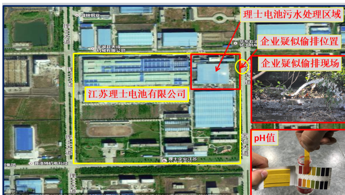
Figure 4. Suspected dumping area of Leoch Battery
