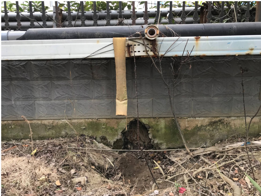
Figure 10.2. The hole in the wall
