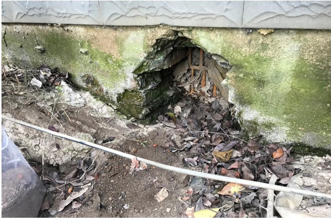
Figure 10.1. The hole in the wall
